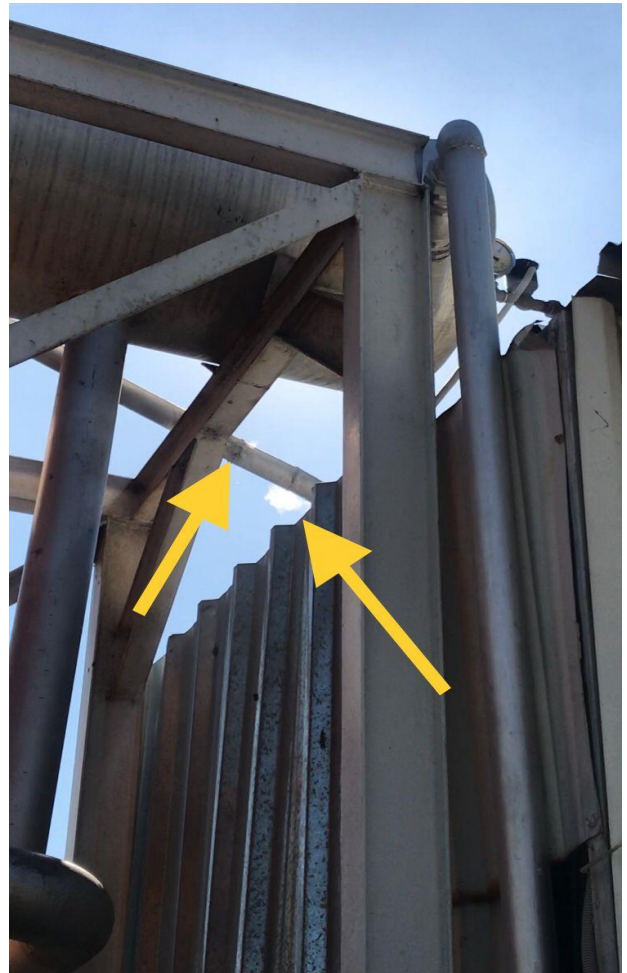
Steam leakage
