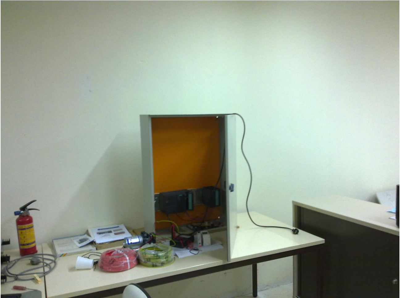
Installation in September 2011 (picture from 21 Nov 2011)
