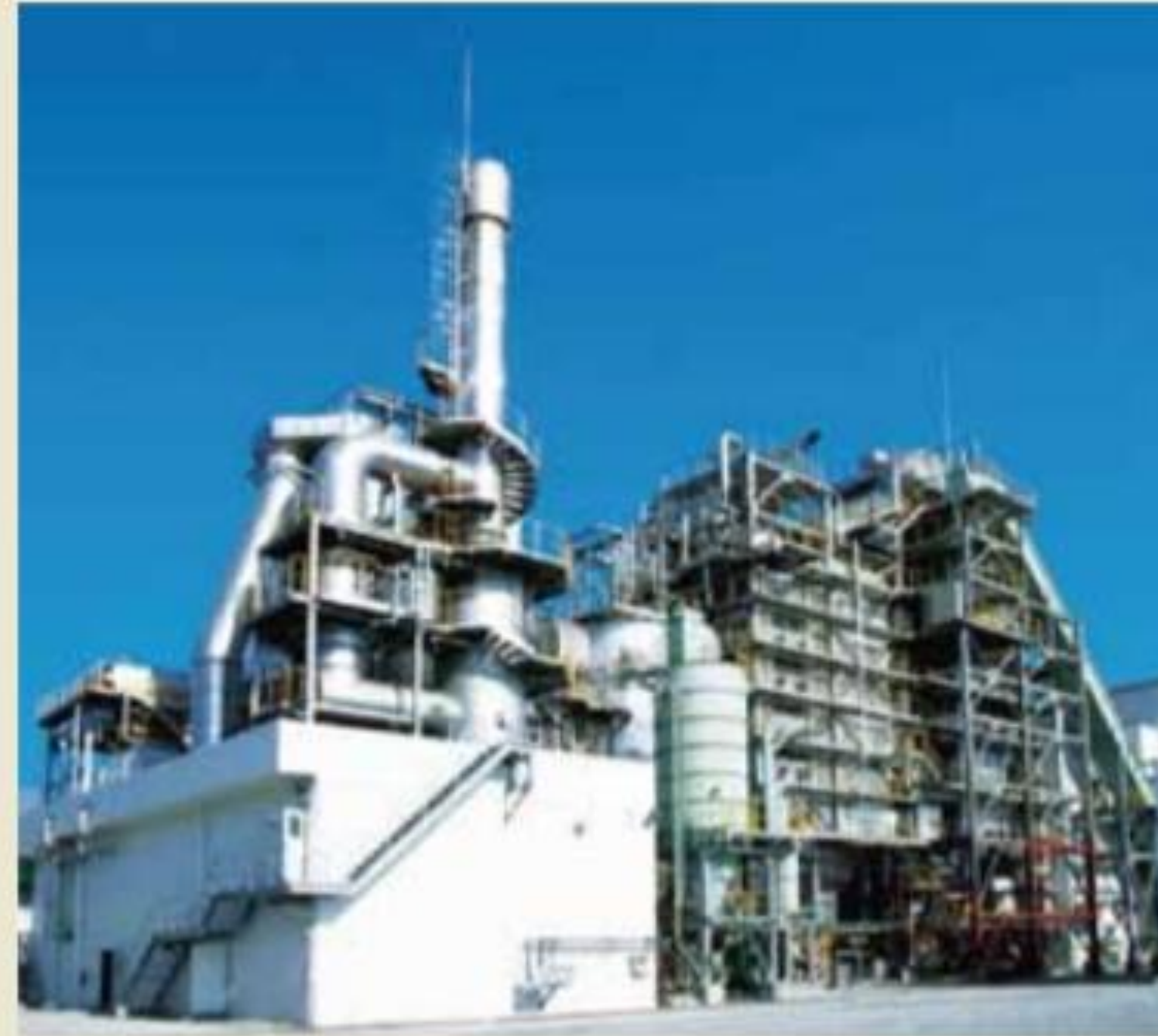
In Thailand, an industrial waste incinerator has been operating from 2006. Its treatment capacity is 100t/day. Source: JFE Engineering Corporation
