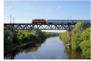
جسر Steel bridge
