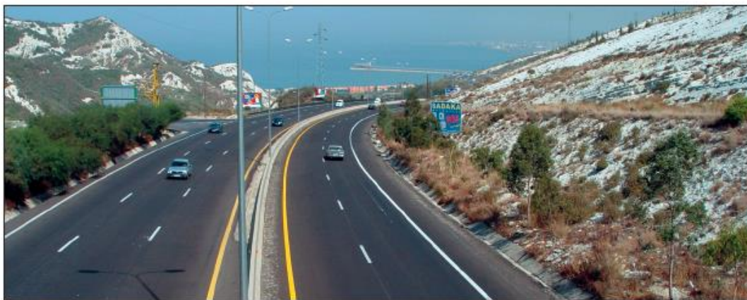
Rehabilitation of Tabarja - Chekka Highway
