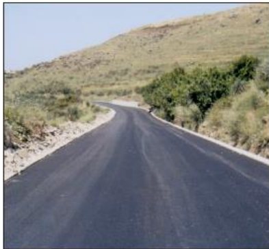
Rehabilitation of different roads in Akkar
