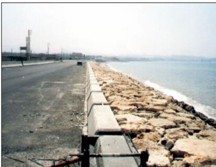
Abdeh-abodyyeh road (Seawall protection and rehabilitation and widening)
