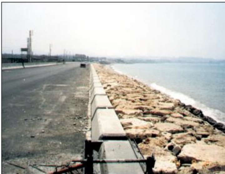
Abdeh-abodiyeh road (Seawall protection and rehabilitation and widening)
