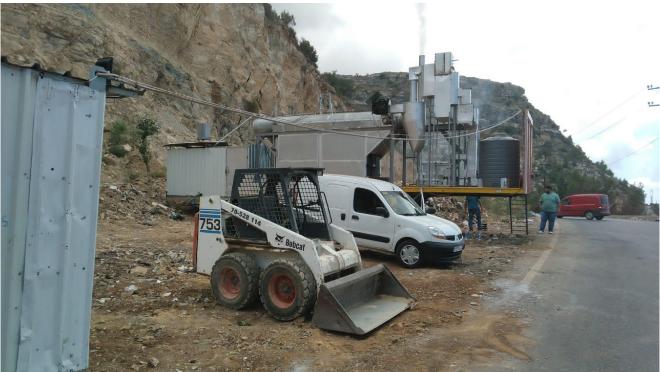
After filtering white smoke can be seen.
