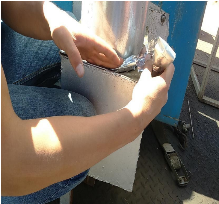
Figure 76: Closing the pores that leak fumes
