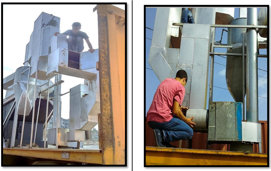
Figure 58:insertion of filter (filter media, large size )
