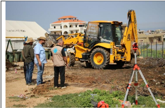
Preparation of ground
