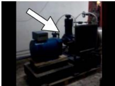
Successful test of turbine
