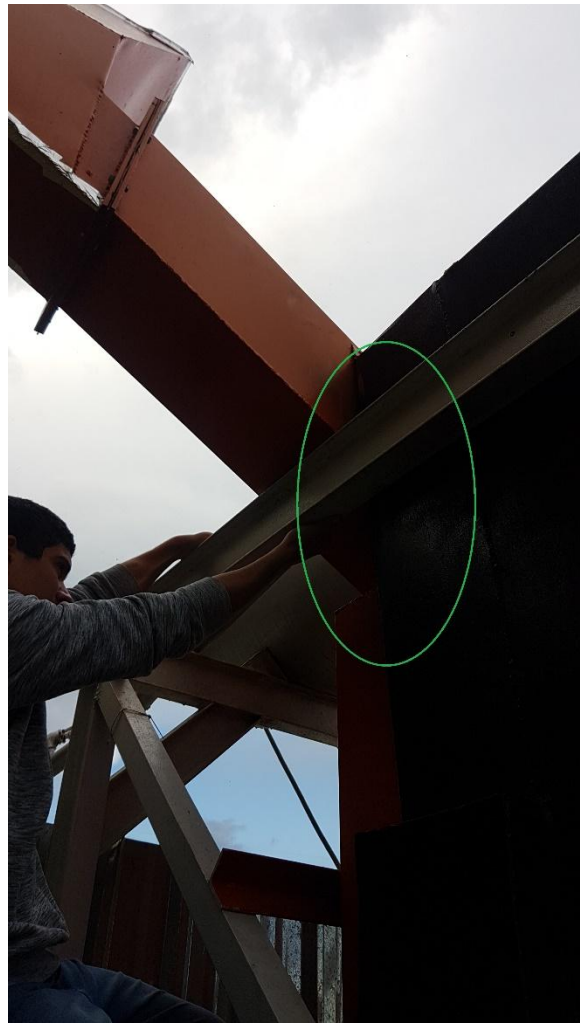
Place 2: garbage entrance
