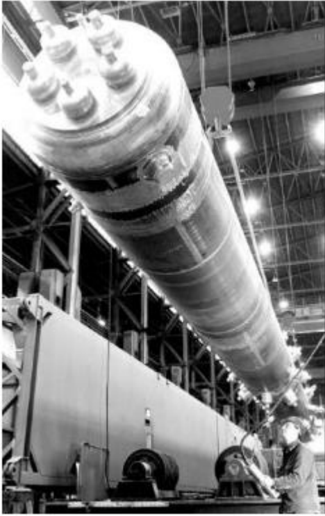
SWHE Installation into Cold Box
