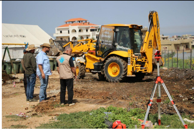
Preparation of ground
