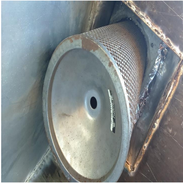
Figure 57:insert of cylindrical media filter after electro filter
