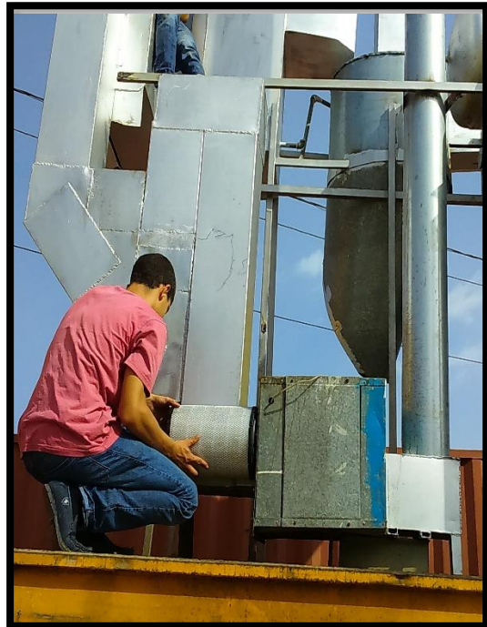
Figure 57:insert of cylindrical media filter after electro filter
