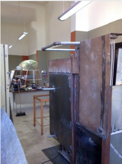
Steam generation unit and overheater unit
