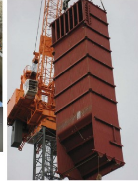
Vaporizer of TEMO-IPP incineration demonstration plant at Ras Nhache/Batroun
