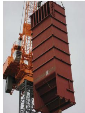
Upscaled vaporizer train element (TEMO-IPP has to be upscaled in such a way) (picture is from Dr.-Ing. M. Franz, "Dampferzeuger", www.axpo-holz.ch/Dampferzeuger.pdf )
