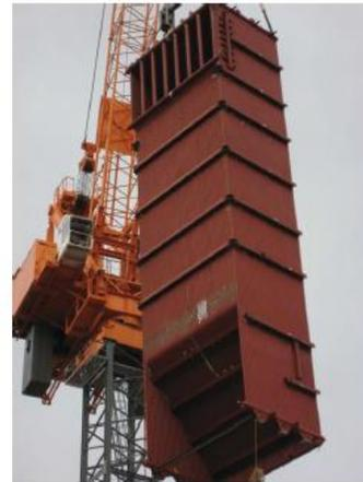
Upscaled vaporizer train element (TEMO-IPP has to be upscaled in such a way) (picture is from Dr.-Ing. M. Franz, "Dampferzeuger", [www.axpo-holz.ch/Dampferzeuger.pdf](http://www.axpo-holz.ch/Dampferzeuger.pdf))
