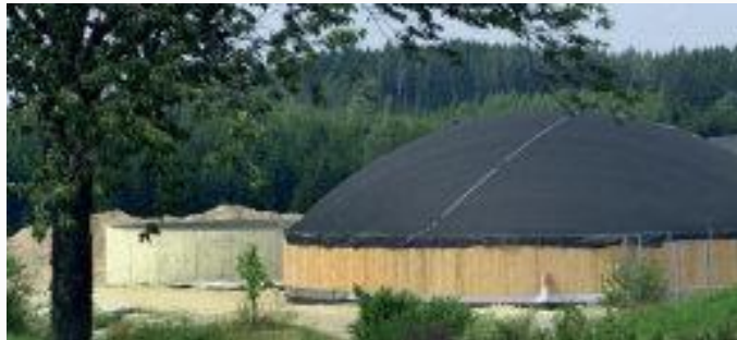
Rubber membrane to maintain the biogas
