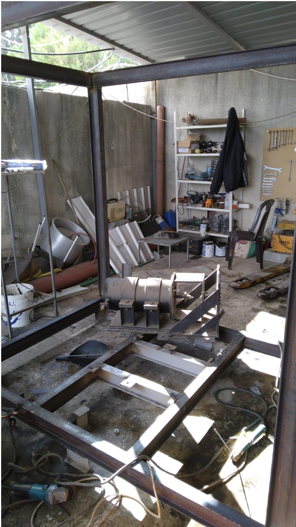
6.4. Gas turbine pieces
