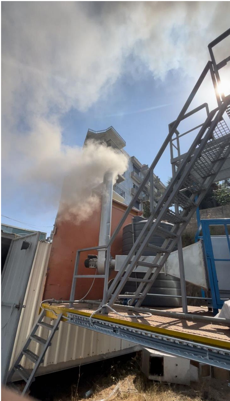
The fire started choking due to water overflow in the scrubber
