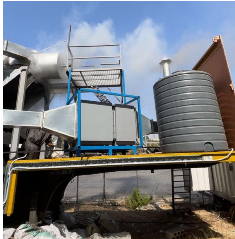
4 water sprinklers added to the scrubber
