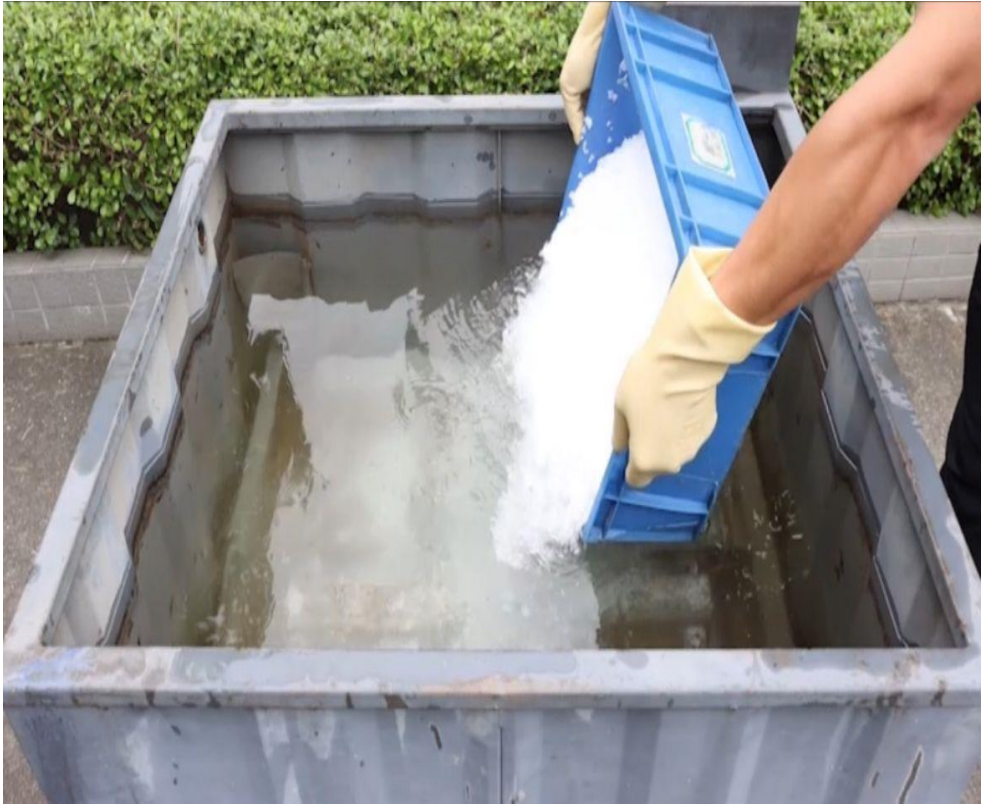
Cleaning Electro-Filter using KLEAN LAND Technique (11.07.2024)
