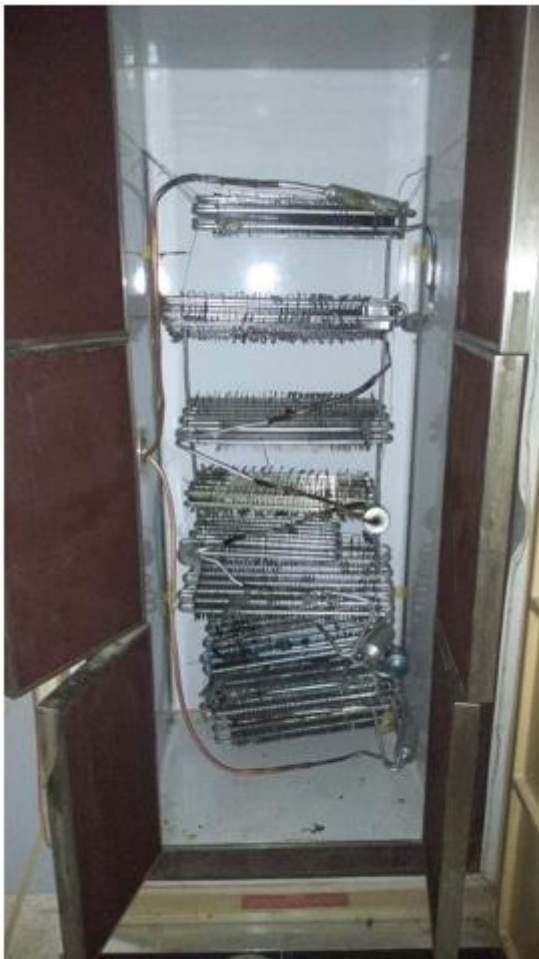
Figure 6. Cooler Tube Implementation
