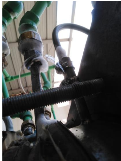
a) Place of leakage of stainless steel
