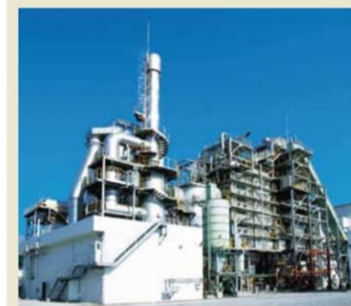
In Thailand, an industrial waste incinerator has been operating from 2006. Its treatment capacity is 100t/day. Source: JFE Engineering Corporation
