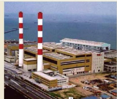
The largest scale plant with the capacity to handle 4,320t/day was built in Singapore in only 38months Source: Mitsubishi Heavy Industries, Environmental & Chemical Engineering Co., Ltd.
