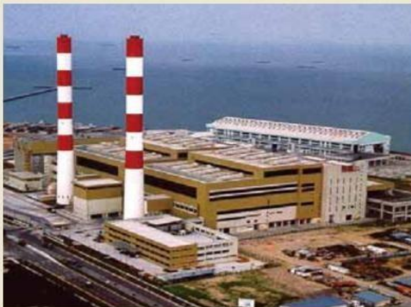
The largest scale plant with the capacity to handle 4,320t/day was built in Singapore in only 38 months Source: Mitsubishi Heavy Industries, Environmental & Chemical Engineering Co., Ltd.
