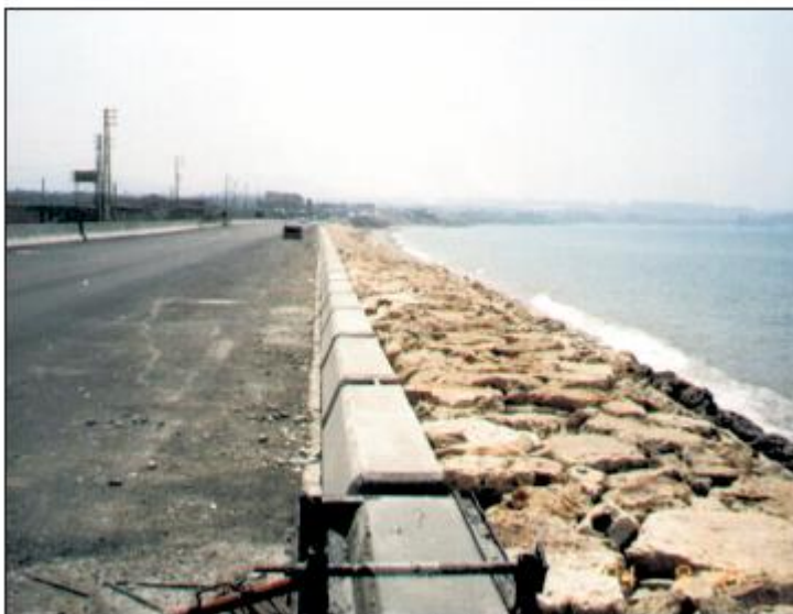
Abdeh-abodiyyeh road (Seawall protection and rehabilitation and widening)
