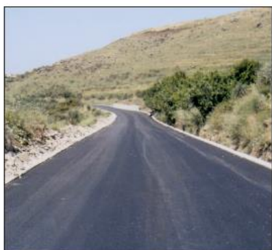
Rehabilitation of different roads in Akkar
