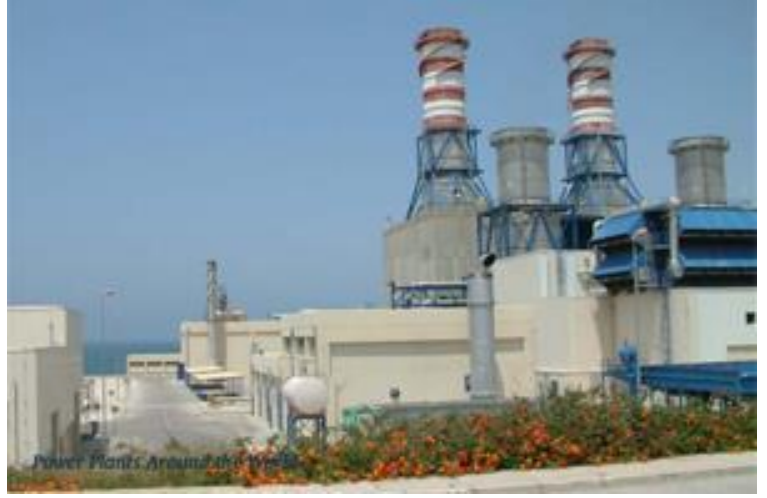
Deir Ammar power plant
