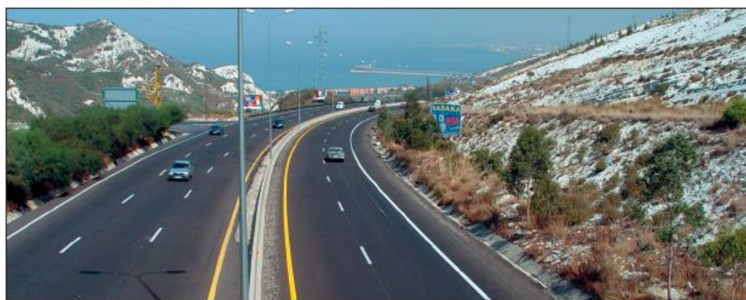
Rehabilitation of Tabarja - Chekka Highway
