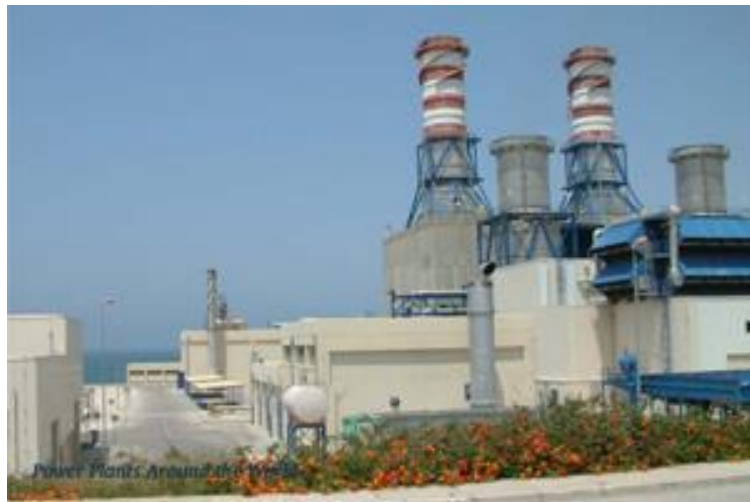
Deir Ammar power plant
