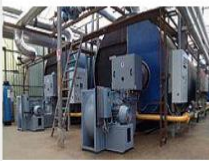
Combustion fan with frequency variator for gas / oil burners
