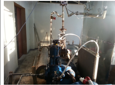
Integration of test rig
