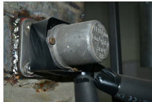
Evaporator automatic level control
