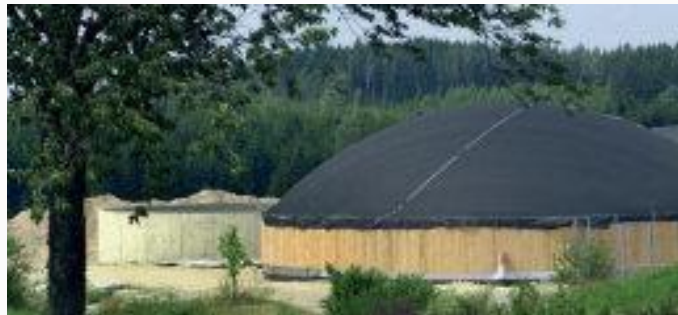
Rubber membrane to maintain the biogas
