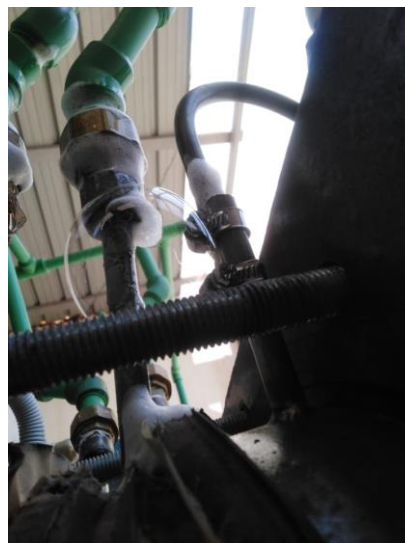
a) Place of leakage of stainless steel
